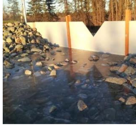
Figure 11: Fall ice depleting dry volume of Spruce detention pond
